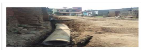
Development of Rigid pavement road network and underground drainage system
