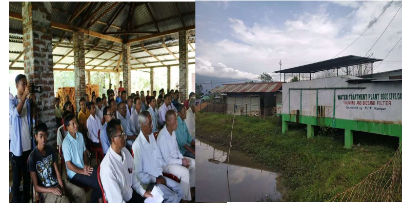
NIT Manipur: 9000 L water treatment plant based on roughing and biosand filters
