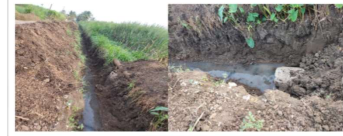
Design and Development (in process) of Sewage Treatment Plant
